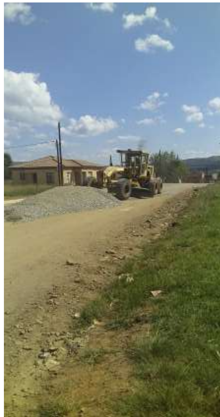
eDumbe Location Road - Ward 3
