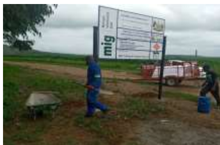
Mdwadlaza Bridge – Ward 1
